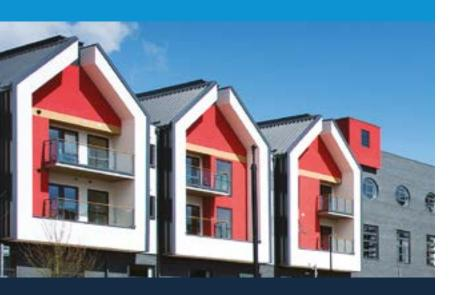
A seamless rendered or brick slip rainscreen system for LSF or timber framed construction.
