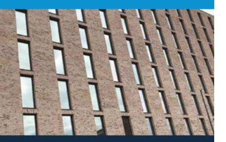
'A' Fire Rated, fast track, mechanically fixed clay brick slip system.
