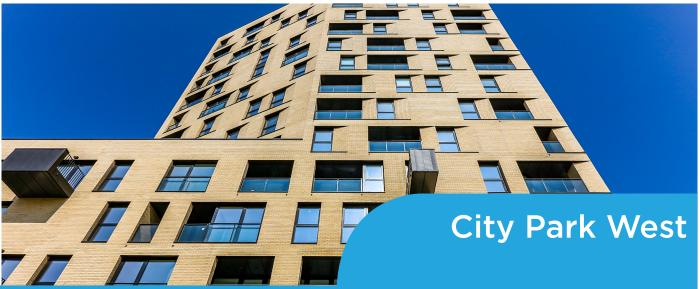
Client: Conneely Facades Limited • Materials: Alucobond Soffit Top Hat Cassettes, Y-Wall, Sector: Residential, Commercial, High Rise • Build Type: New Build Aluminium Support Frame
