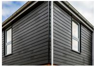
RCM were asked to supply their Supertech Weatherboard for the exterior of the different types of houses, ensuring an individual finish for the different house types.
