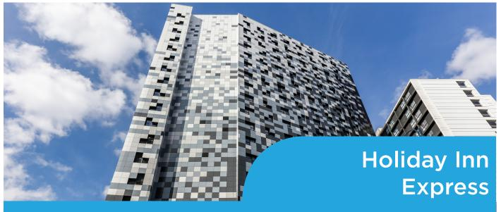
Client: John Sisk and Son • Materials: Vitrabond ACM, Aluminium Facade Support Frame, Traspe HPL Sector: Hotel and Leisure • Build Type: Modular Precase Concrete
