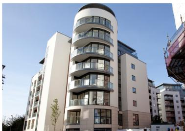
The works at Kew Bridge, which is of concrete frame construction using lightweight steel walling and cement particle board, started in the May 2013, where Stanmores worked very closely with SPSenviowall to install 10,634m<sup>2</sup> of render amongst the nine blocks.
