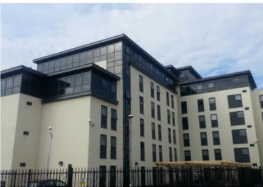
This is a fast track construction of student accommodation in the centre of Cardiff. The frame of the construction is cast concrete with a lightweight steel infill.
