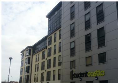
120mm of white EPS with mineral wool fire breaks has been fitted external to the frame, generating a U-Value of 0.22W/m<sup>2</sup>K.
