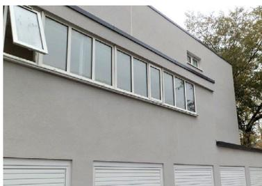
Carried out over the duration of eight months, P&P and SPSenviowall successfully installed 3,500m<sup>2</sup> of 90mm grey EPS insulation, which provided the residents with a more comfortable living environment by improving the thermal performance and in
