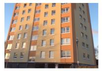
Raeburn Heights is a 16 storey residential high rise block in Glenrothes, Fife which has recently undergone a £350,000 refurbishment to install external wall insulation and other energy efficiency measures.
