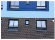
The 60 year old buildings, constructed with rendered concrete wall panels on a concrete frame, had poorly insulated solid walls.
