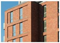
Eye-catching, fire-safe Cavity System 2 and SpeedySlip Brick Façade for Wheatstone House, London
