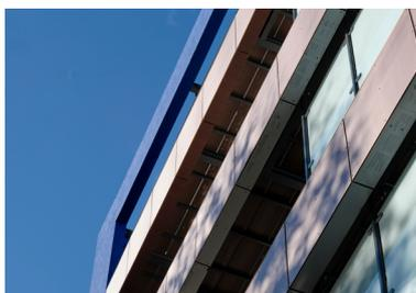
LB&F Façade Specialists expertly installed SPSenviowall's Cavity System 1 with a white silicone render complemented with RCM's Rockpanel FS-Xtra as part of the façade package supplied to the project.
