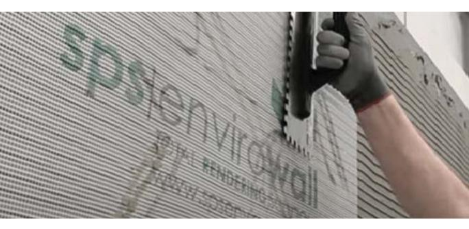
Our reinforcement mesh is the unsung hero of the render-only or EWI system. The mesh provides reinforcement and stability to the render, thus creating a perfect base for the subsequent application of an **SPS EnvirowalI** finish product.
