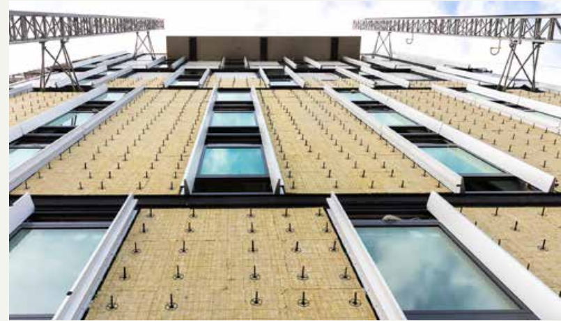
A stone wool insulation effectively works against temperature and noise
