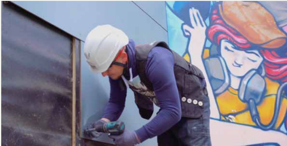
Easy dismantling of Rockpanel boards
